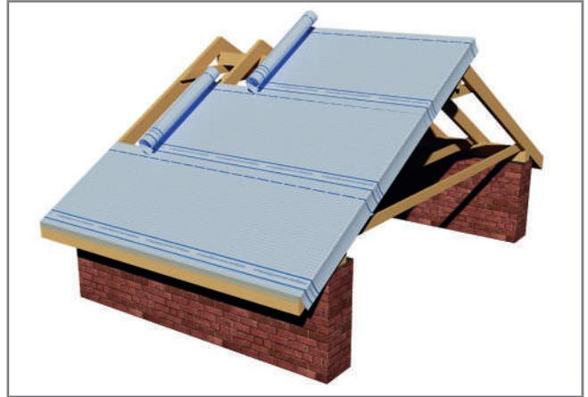
Fig 8.2.1 Membrane installation
